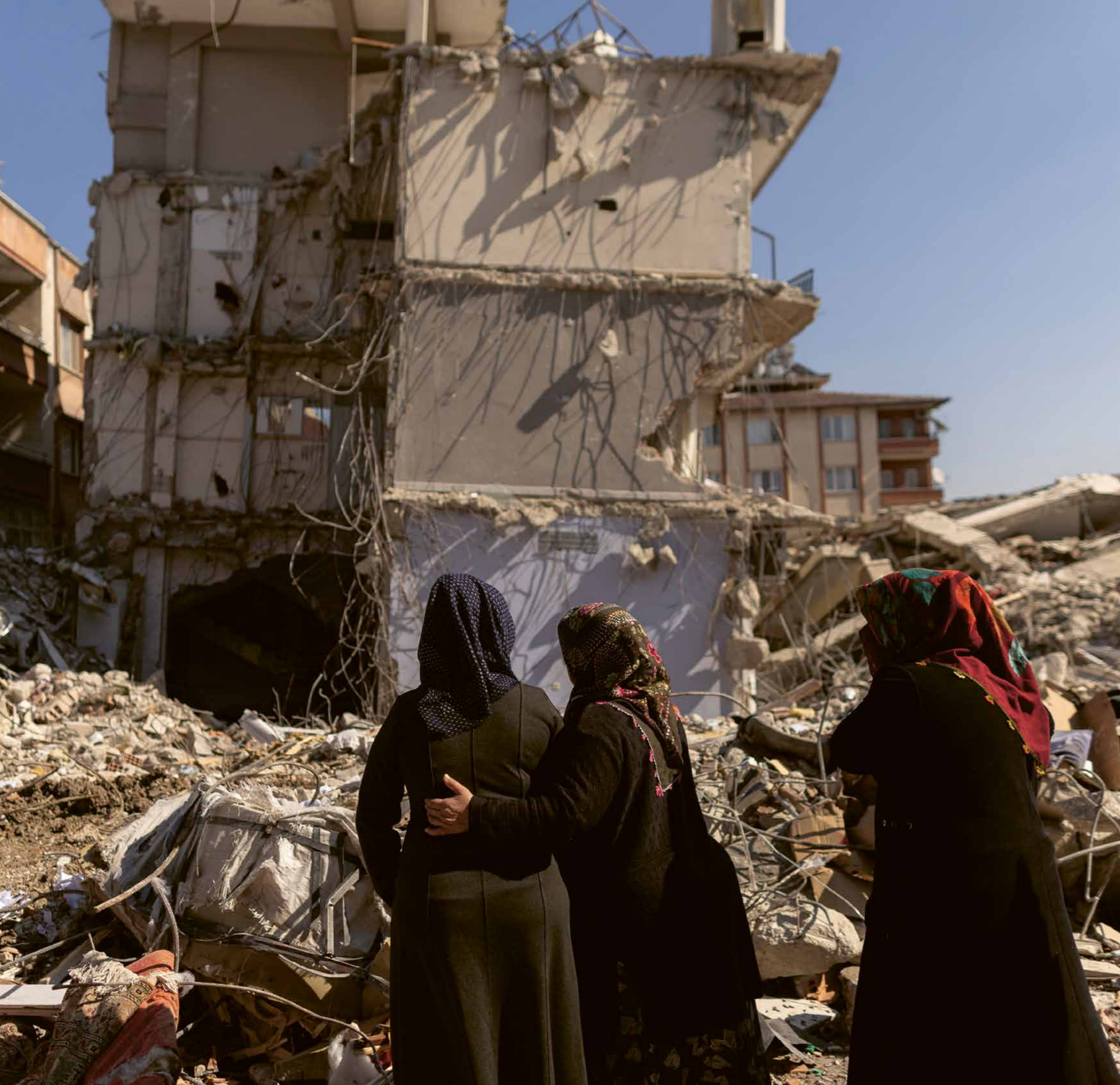
Women look at what is left of their home following the deadly earthquake in Hatay Province, Turkey. © Reuters/Eloisa Lopez/2023
