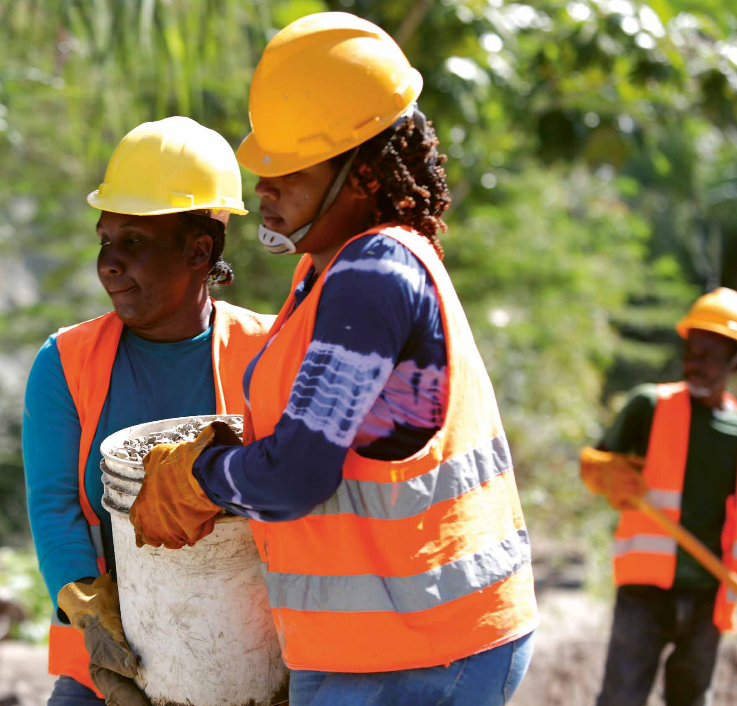
Construction work in Haiti's Nord-Ouest Department. © UNOPS/2025
