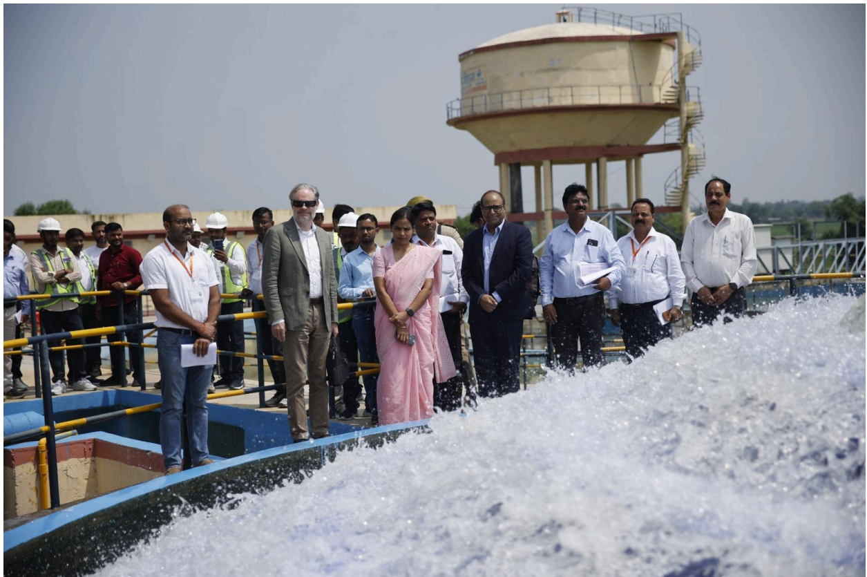
Ambassador and senior government officials at the Water Treatment Plant
